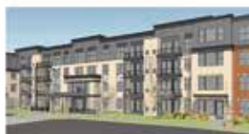
Millberry Apartments Affordable Multifamily Housing 121 Units | St. Paul, MN $17,016,000 HUD 221(d)(4)
