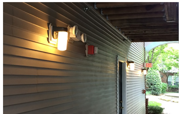
Interior Hallway-Installed LED Lights
